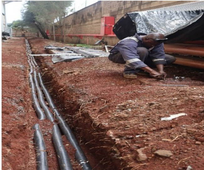
Photos of HVAC project in progress in the warehouse.
