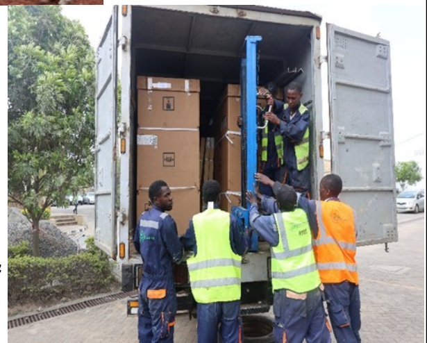
VRF outdoor units being delivered & electrical cable layout respectively.
